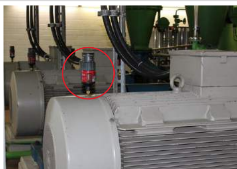
Electric motor bearing lubrication
